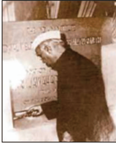
Pandit Jawaharlal Nehru laying the Foundation Stone of the Academic Block, 1958
